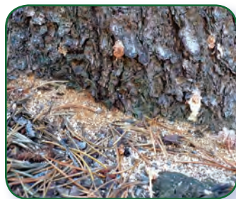
Pitch Tubes and Boring Dust
