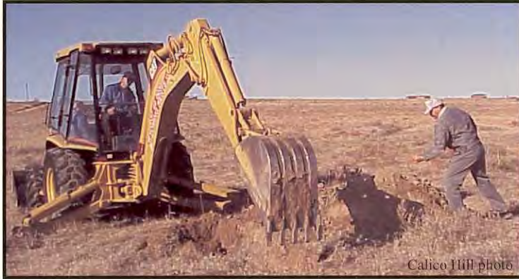
Exploratory Trench—Health Department Inspection
