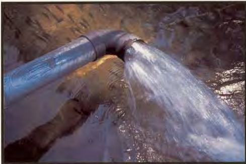
The welcome result of successful water well drilling.
